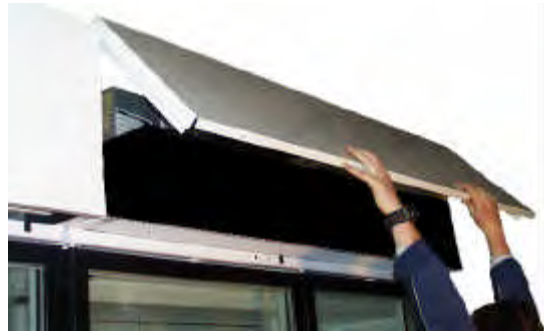
Figure 12: Solid Pelmet Removal
