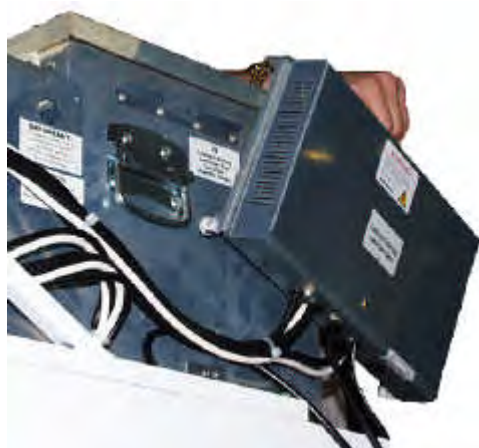
Figure 20: Junction Box Removal
