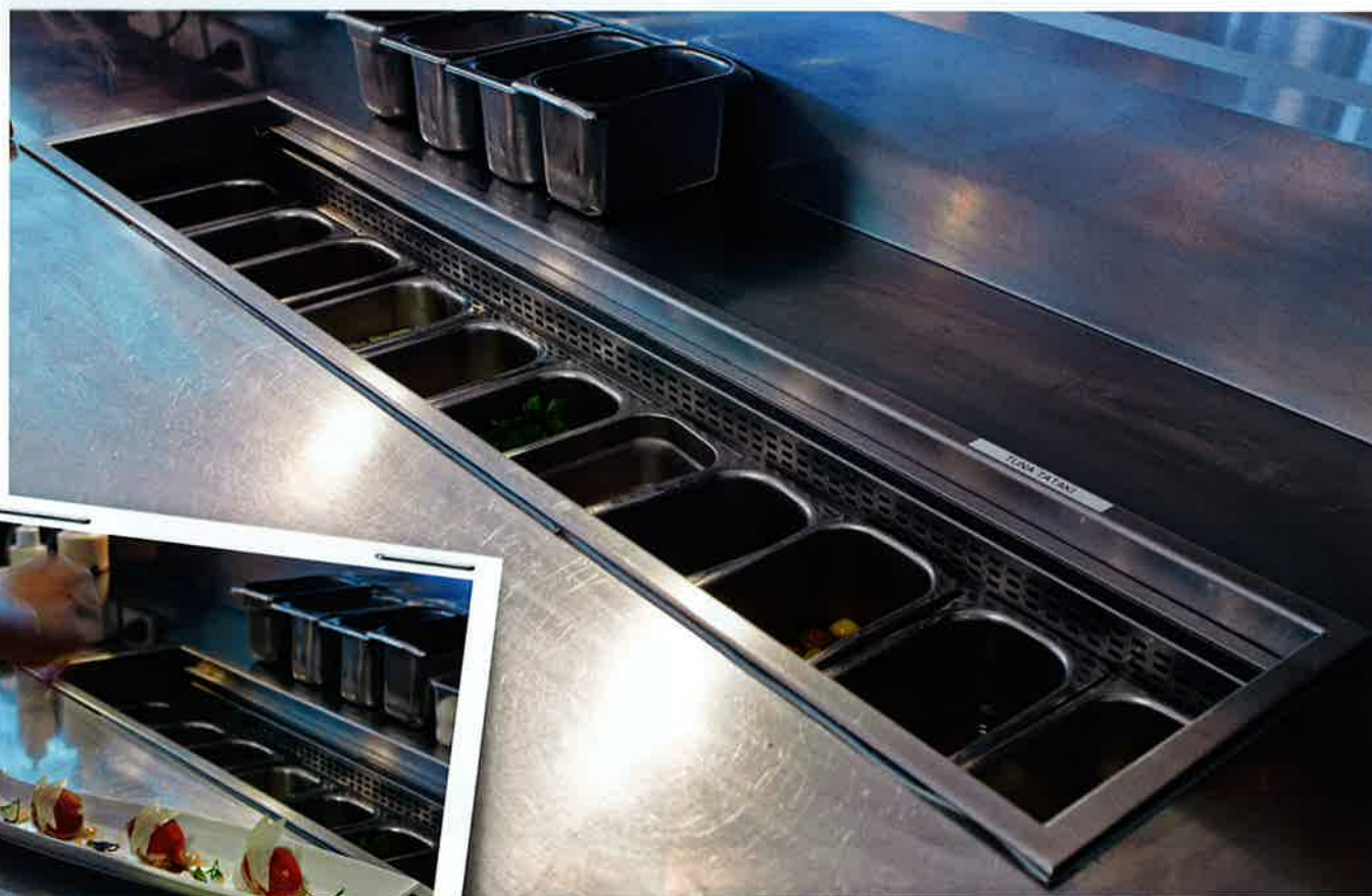
Chef Maunder has easy access to the new recessed chilled wells in one of the service lines as he prepares a fresh tuna tataki dish. The wells prevent him from going back and forth to the fridges.
